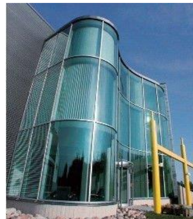
Fig. 1: Curved glass plates as curtain wall
