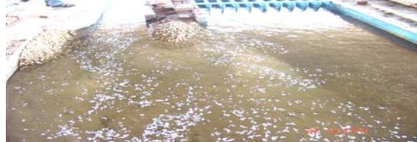
**Photo 4.** Flow Currents D.S. Barrage using 20 m Long SGW ( $Q_{min}$ )
