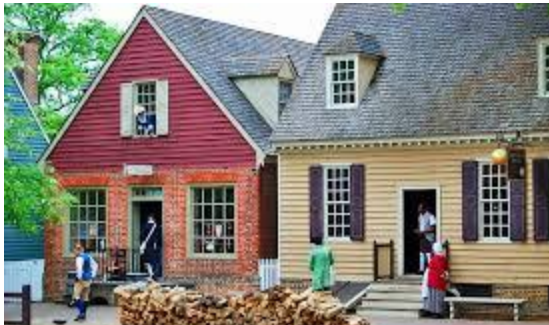
Fig.-19. shows the large areas of external openings and using of transparent glass in the windows
