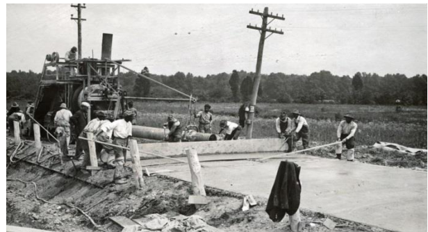
Fig.-10. Construction of the Colonial Parkway
