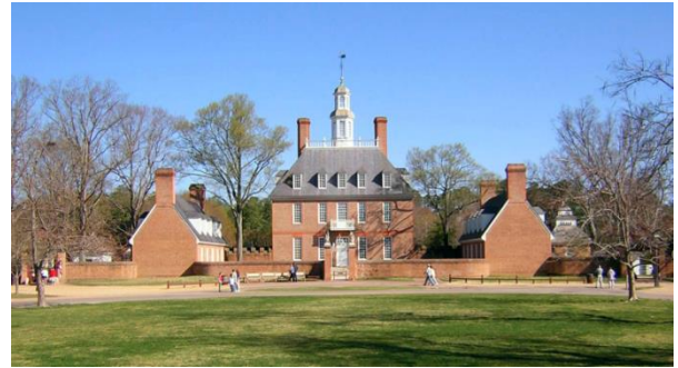
Fig.-25. the proportion of open spaces to the mass allowing permanent and sustained air movement
