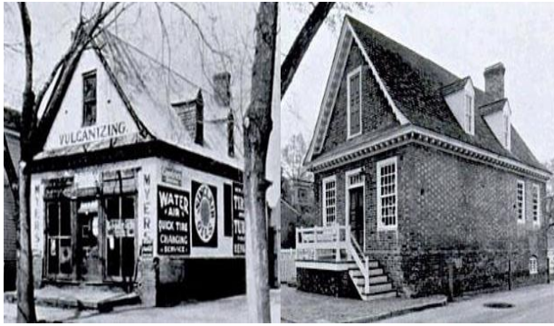
Fig.-23. The Prentiss Store showing the re-adjustment of existing structures during the restoration
