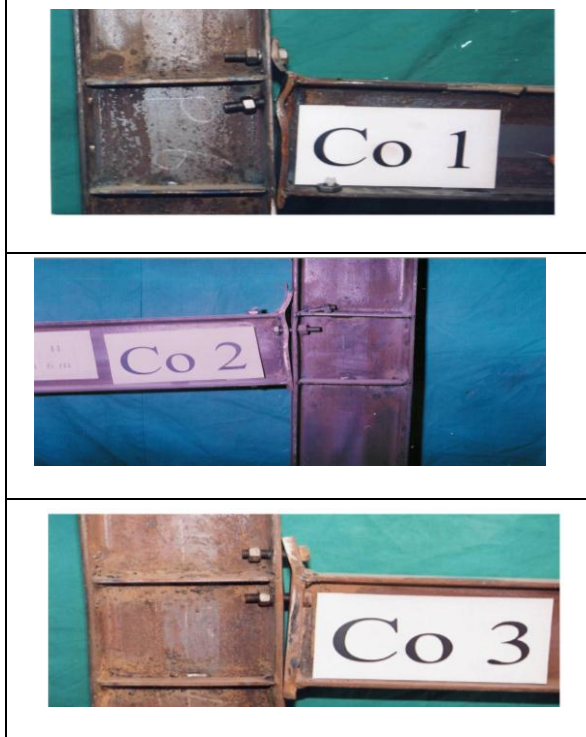
Fig. (25): Modes of Failure for the tested connections (Co.1, Co.2 & Co.3) in the group I
