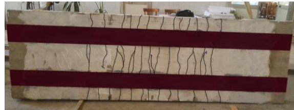
Fig. 23: Cracks pattern for S2ST3 at p=200 kN
