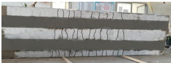
Fig. 19: Cracks pattern for S2G4L at p=155 kN
