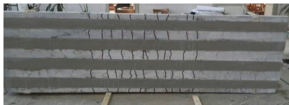
Fig. 17: Cracks pattern for S4G2L at p=145 kN
