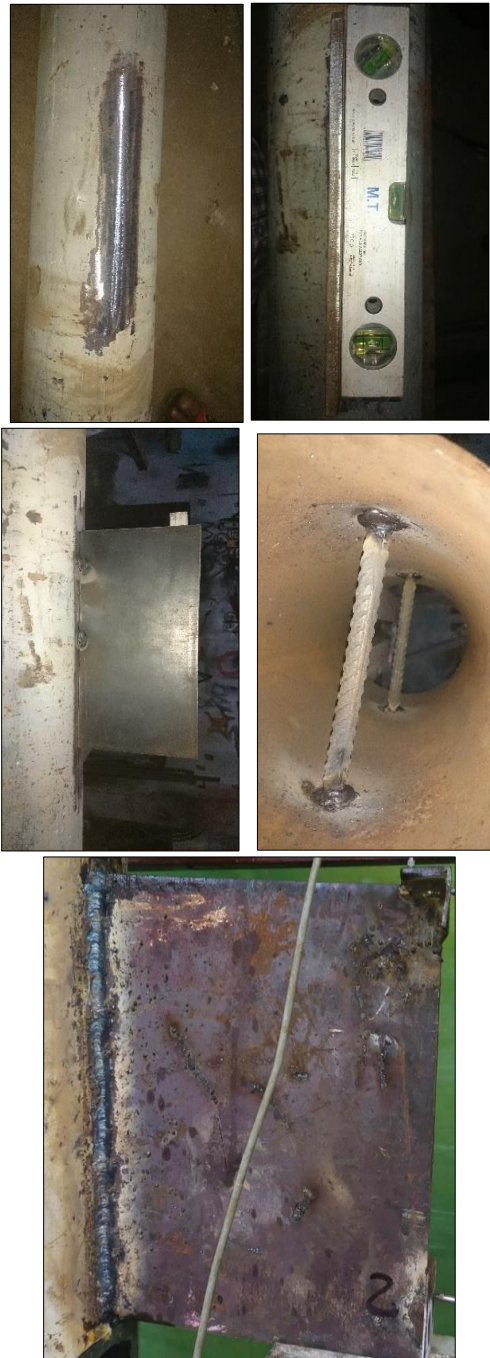
Figure 4- preparing of connection
