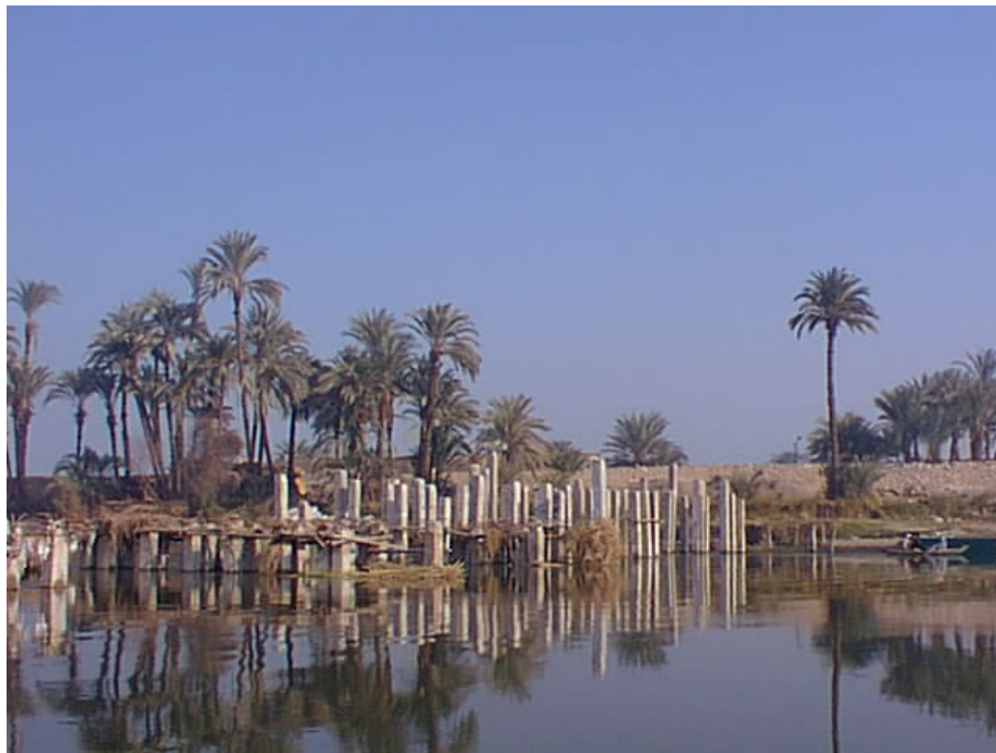
Fig.1 Driven piles of the bridge in Upper Egypt
