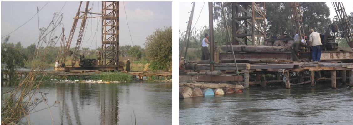
Fig. 11 Platform setup used to drive piles of bridges across water courses
