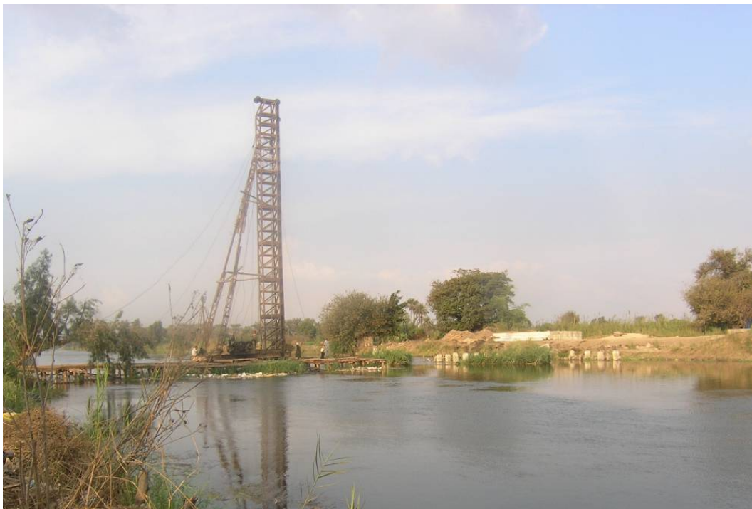
Fig. 3 Driven piles of the bridge in the North East of Egypt
