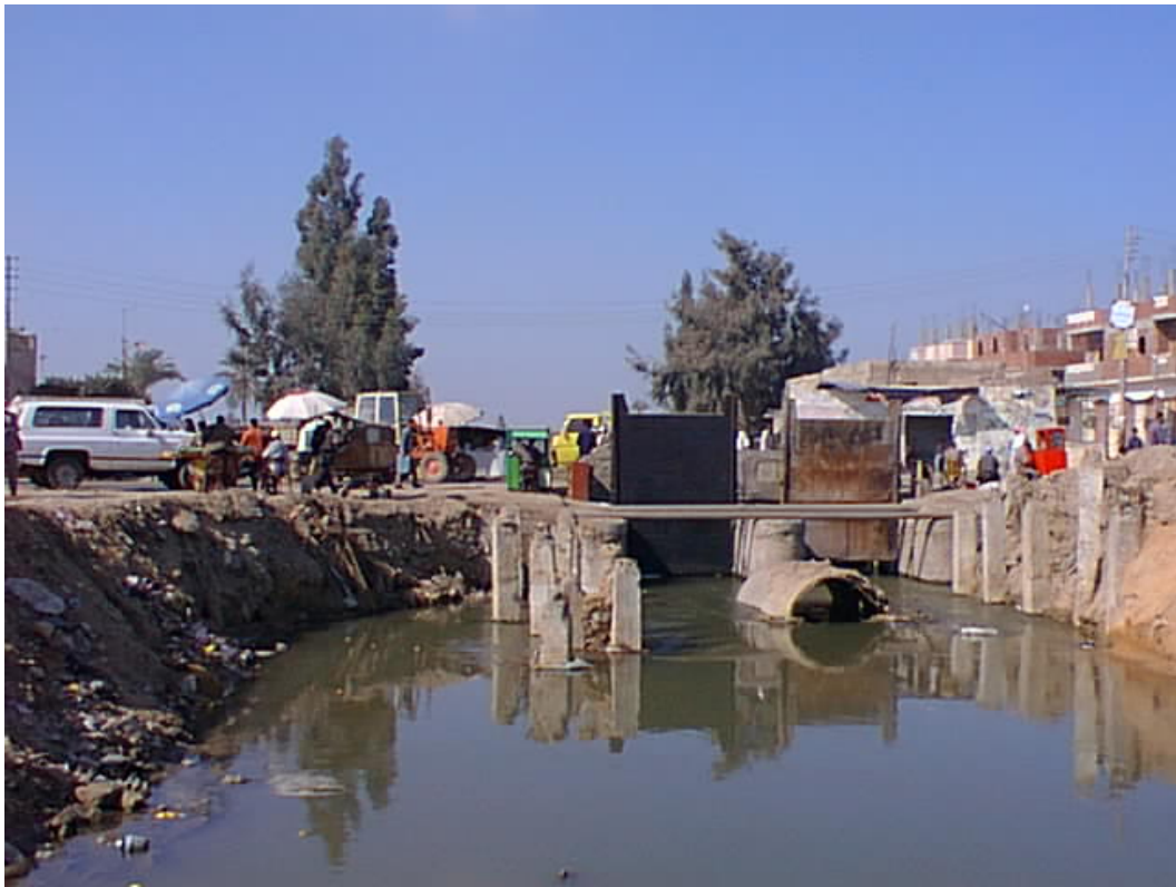
Fig. 2 Driven piles of the bridge in North West of Egypt
