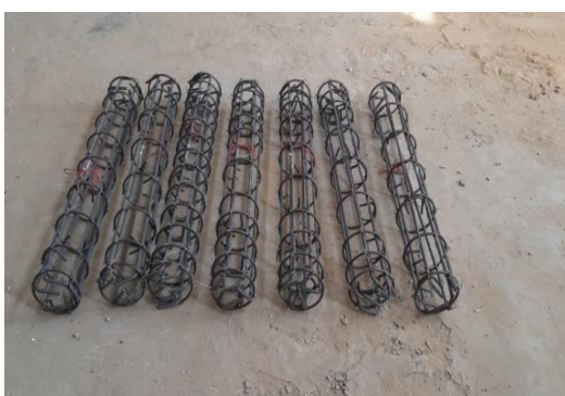
Figure 4 – Steel cages for group (B).
