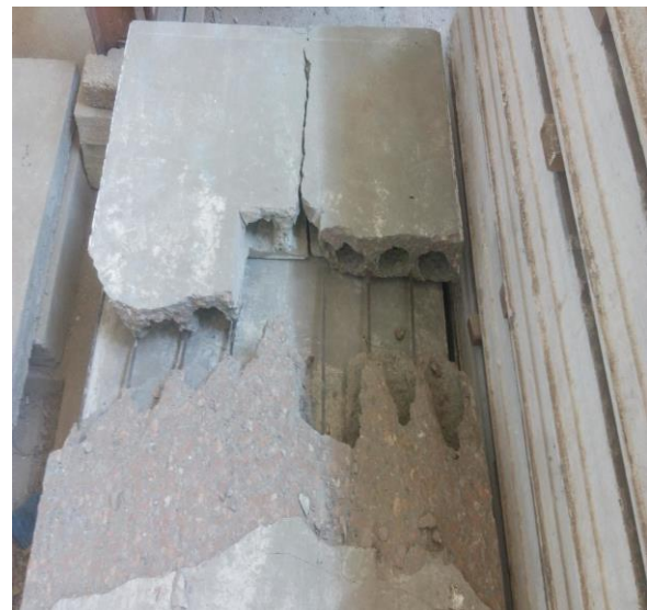
Fig. 13: Failure and Cracks pattern for PPHCS3
